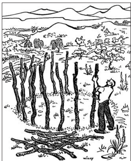
Starting the first 'Residence' using wattle-and-daub building method.
